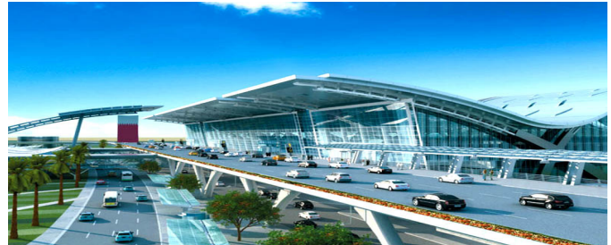
View of the Hamad International Airport (HIA), recently listed as one of the Top 10 Best Airports in the world.
